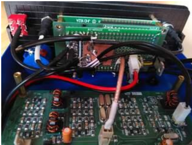
Figure 11. Front panel interconnect board and associated mess wires
